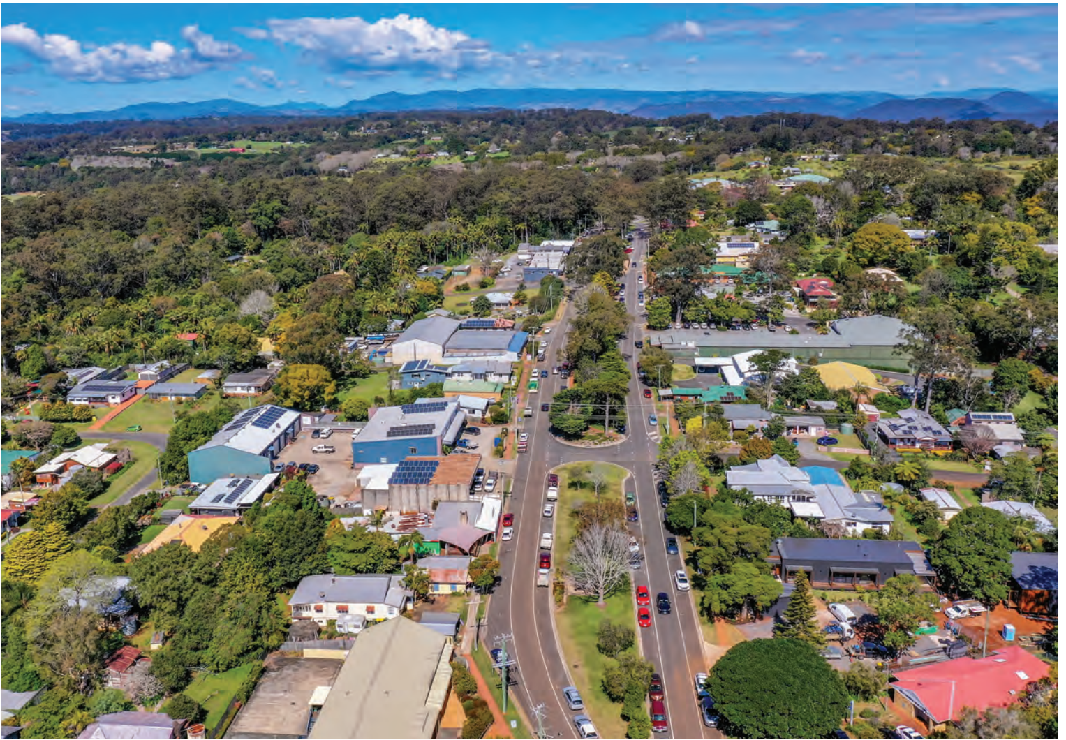
A spectacular springtime view of North Tamborine's Main Street, looking south towards Lamington National Park and the Border Ranges. The police station is at bottom right; other prominent buildings easily visible are the Main Fitness Gym (middle left) behind Tyrepower, Mitre 10 and (middle right) the old IGA building. Photo: G. Ellen
