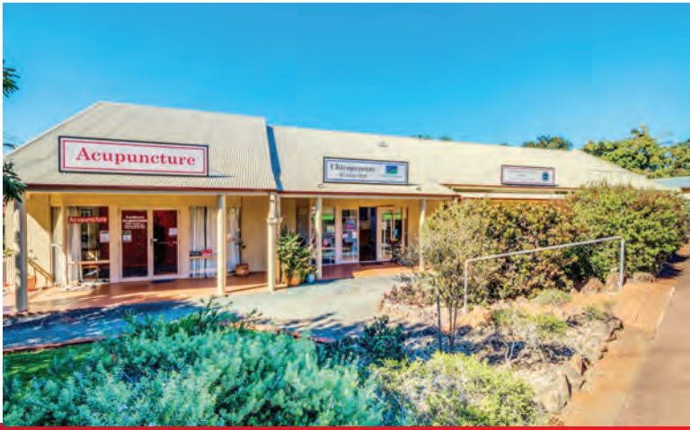
Shop 4/49 Main Street, Tamborine Mountain
