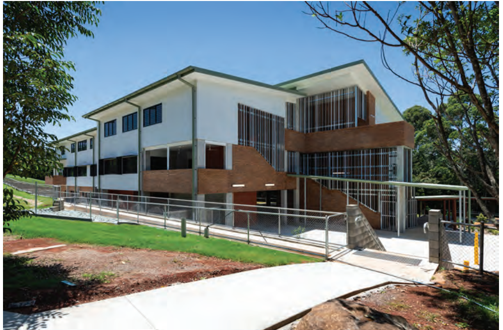
The new $11.3 million learning centre at Tamborine Mountain State High School
